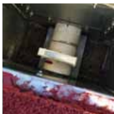
Internal gate valve allows for quick and easy drainage of the water jump pit.
