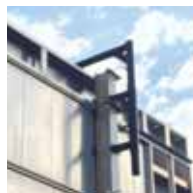
Custom mounting bracket anchors netting on SNS-MBS model.
