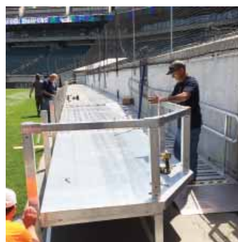
Individual platform components were manufactured in AAE's shop and delivered for on-site install
