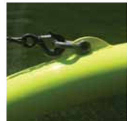
Welded bracket permits a winch and cable to mechanically raise and lower the entire goal.
