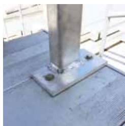
Aluminum mounting bracket secured in four locations to existing platform.
