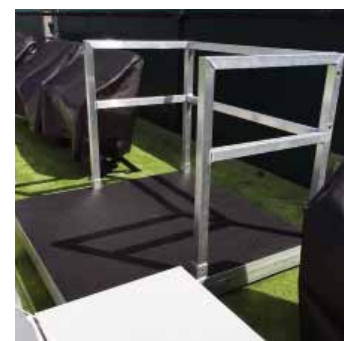
Independently suspended camera platform stabilizes video equipment to avoid potential tremors from people walking on endzone platform
